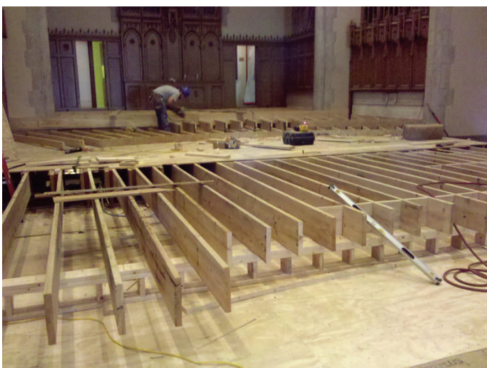
New Chancel structure
