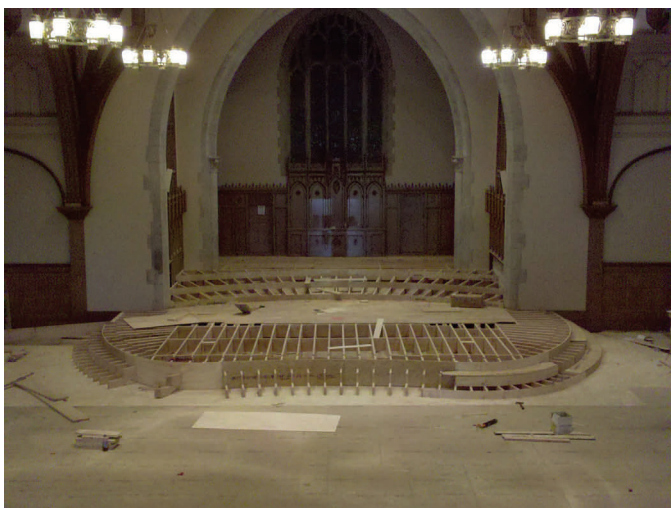
Chancel as seen from the East Avenue balcony
