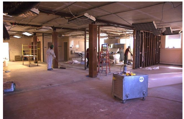
Celebration Center Stripped, Kitchen being demolished
